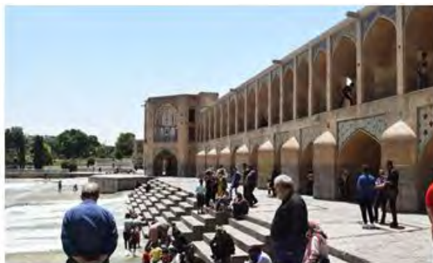
Fig. 2: A side view of the Khaju Bridge; Isfahan City
