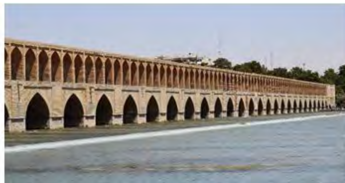
Fig.1: Allahverdi khan bridge
