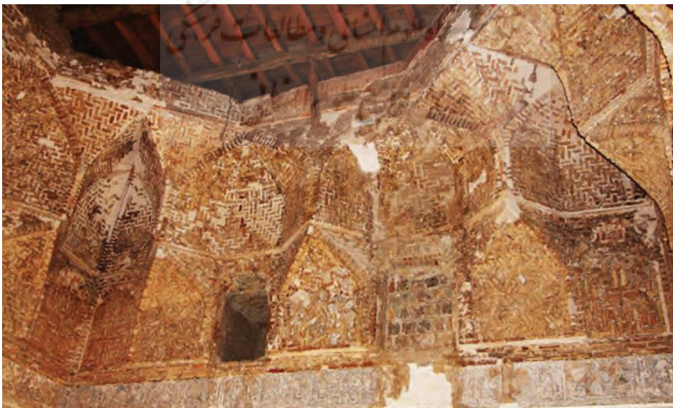
Fig. 7: Marand Mosque; an interconnected set of concave units in the transition zone.
