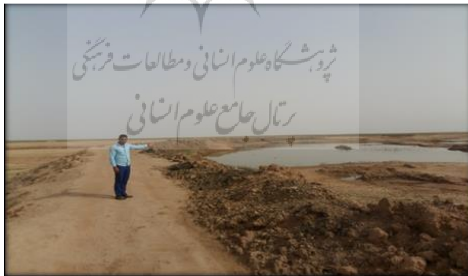
Figure 1. Shows the earth dams built on the valley basin
