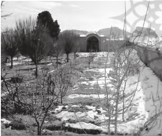
Fig. 8. View of a manor on Hirmand farmstead
