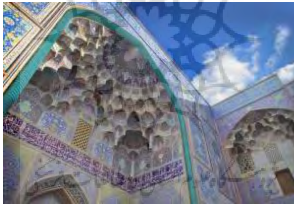
Image 12- The muqarnas decoration of the entrance way of Sheikh Lotfoallah Mosque ( www.tripyar.com )
