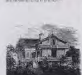
Figure 6.14 The 'Cutter' building, designed by Kirtland Cutter (1810-1870), and built by Matthews in the 1840s.
