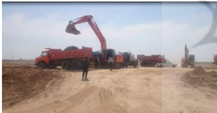
Picture 3 Excavation from natural environment (Location: A connecting road, Ahvaz) Source: (Author)
