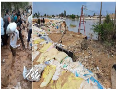
Picture 5 Levees made of plastic materials and clay Source: (Unknown)
