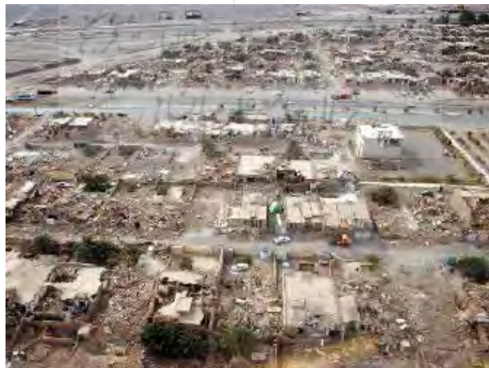
Figure 4- Severe urban tissue damage in the earthquake in Bam
