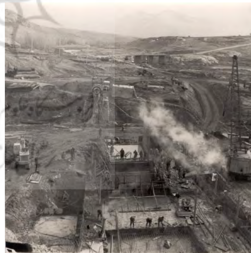
MAHABAD PROJECT Spillway - Bucket Bottom Outlet Side
