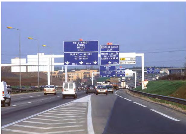
A4 Highway - Marne-la Vallée
